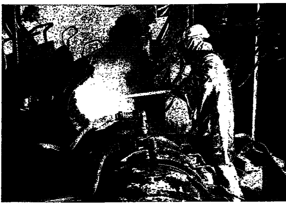
The Bingham Canyon smelter-refinery project should be operating at full capacity by 1997
